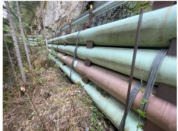
Steel pipe and cable leash facing
